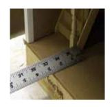
Measuring the stairs in the standard cutout shows a run of about 7"... the hole will have to be moved  $2^{1/8}$ " frontward to give 5/8" clearance behind a divider door cutout
